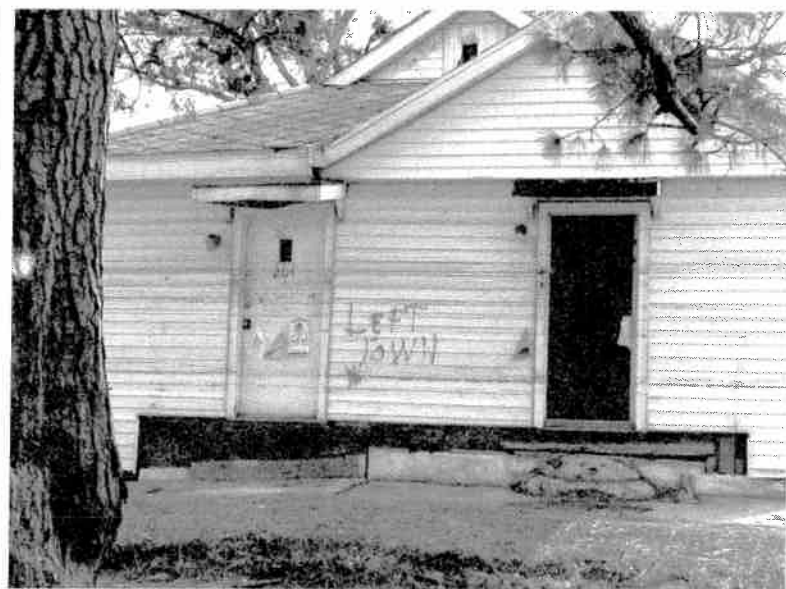
High water lines.
